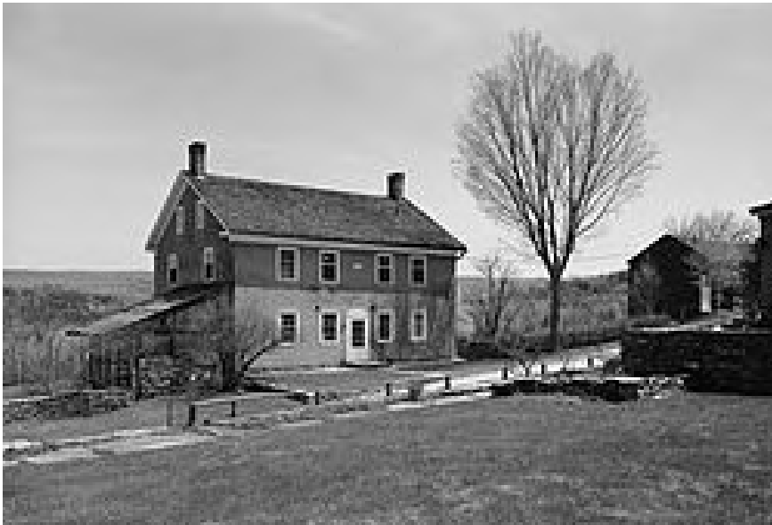
Building in Tyringham Shaker Settlement, Photo courtesy of the Library of Congress
